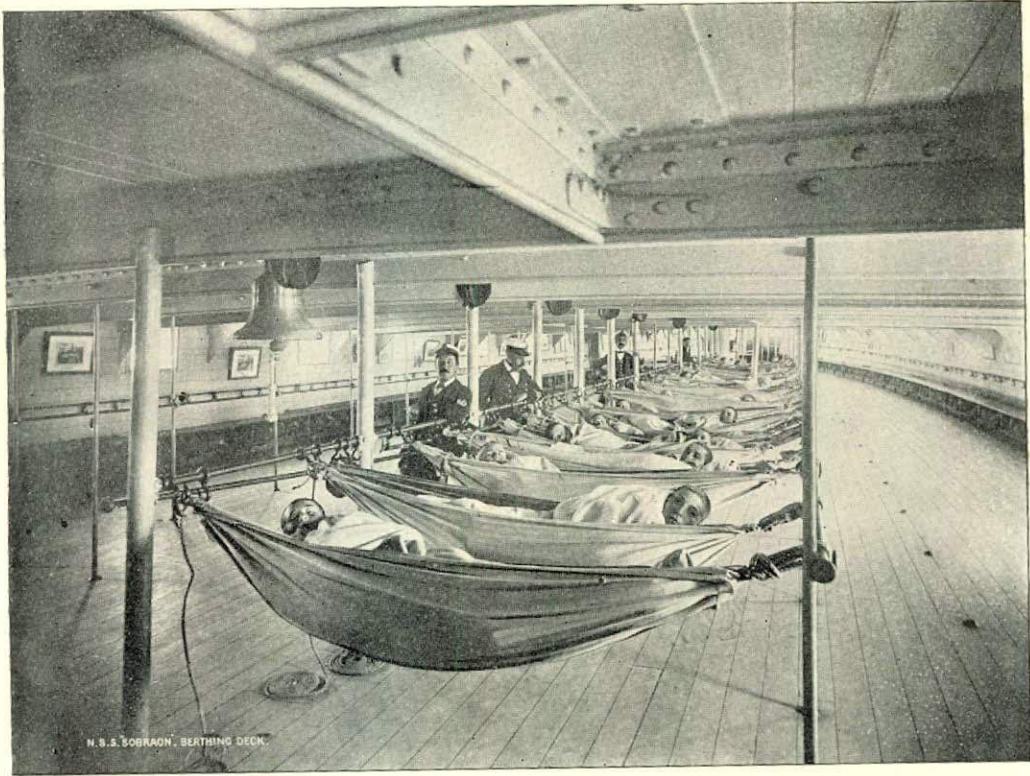
N.S.S. "SOBRAON."—BERTHING DECK.
