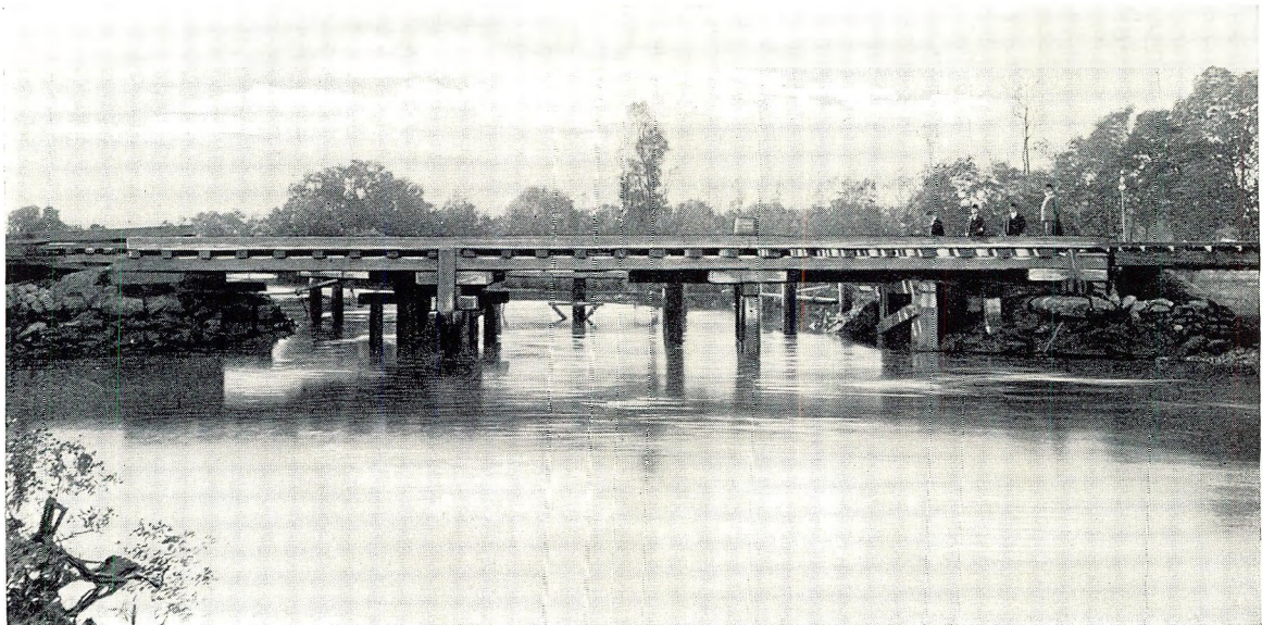
OLD TIMBER BRIDGE OVER IRONBARK CREEK.
