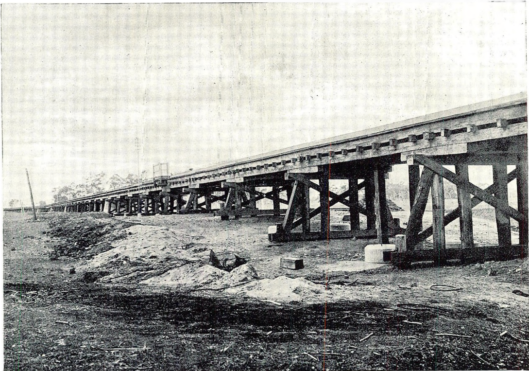
OLD WOODEN VIADUCT.
