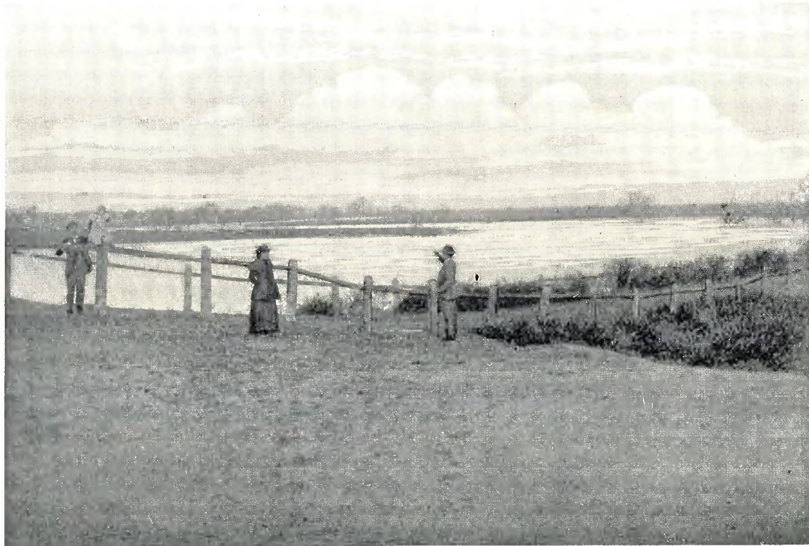
URANA CREEK—VIEW LOOKING UP STREAM SHOWING WATER CONSERVED BY TOWN DAM.
