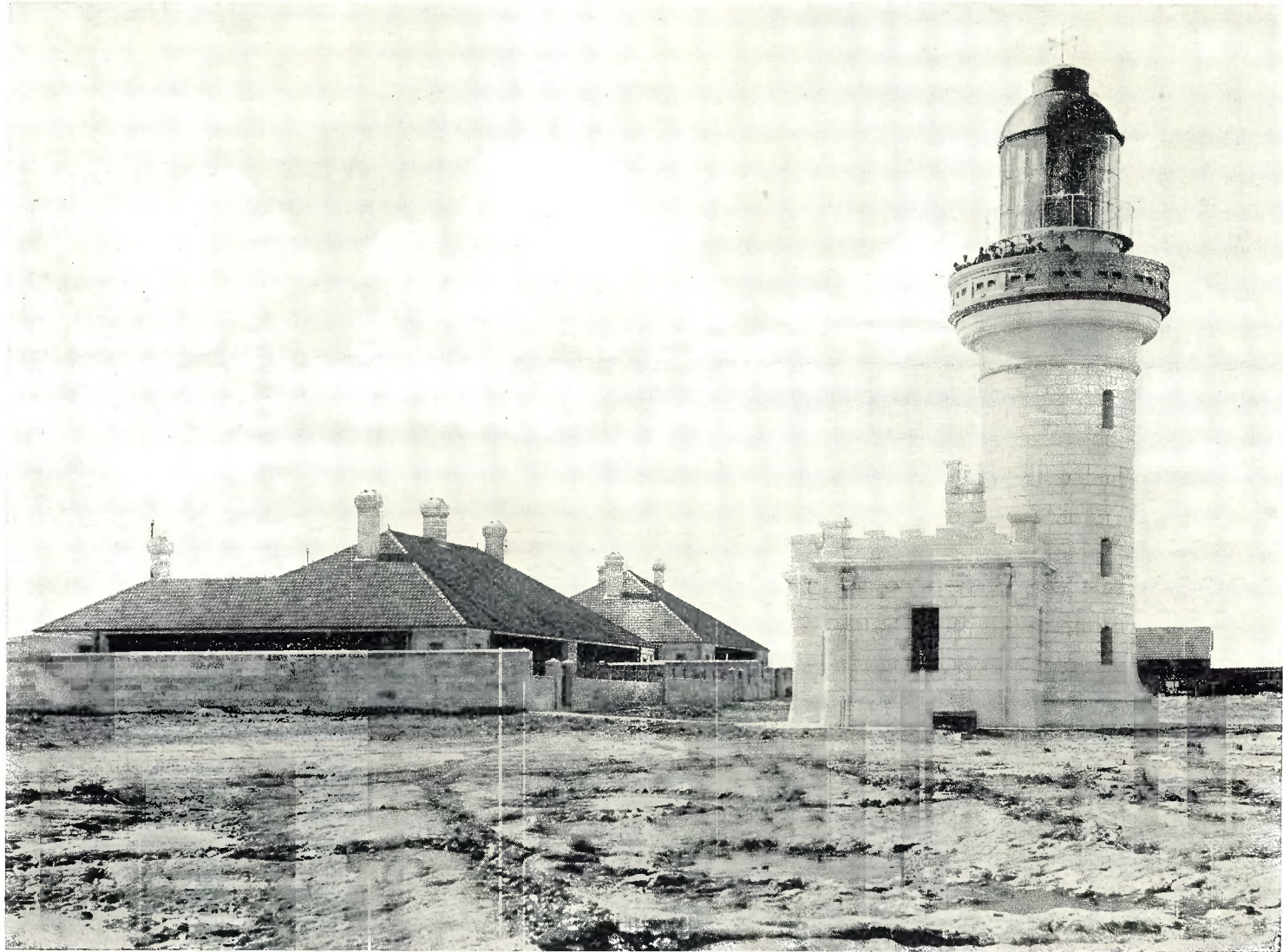
POINT PERPENDICULAR LIGHTHOUSE AND QUARTERS NORTH HEAD, JERVIS BAY.
