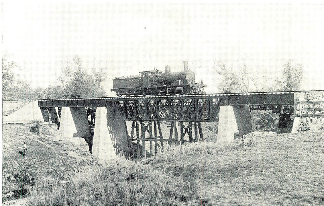
STEEL BRIDGE OVER SALTWATER CREEK. (Old timber bridge at back.)
