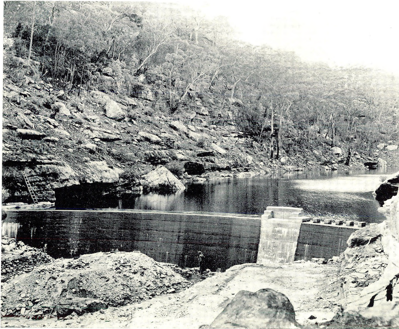
PICTON WATER SUPPLY—DAM ON BARGO RIVER.
