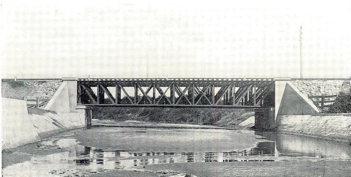
NEW STEEL BRIDGE OVER STYX CREEK. Span 72' 10".
