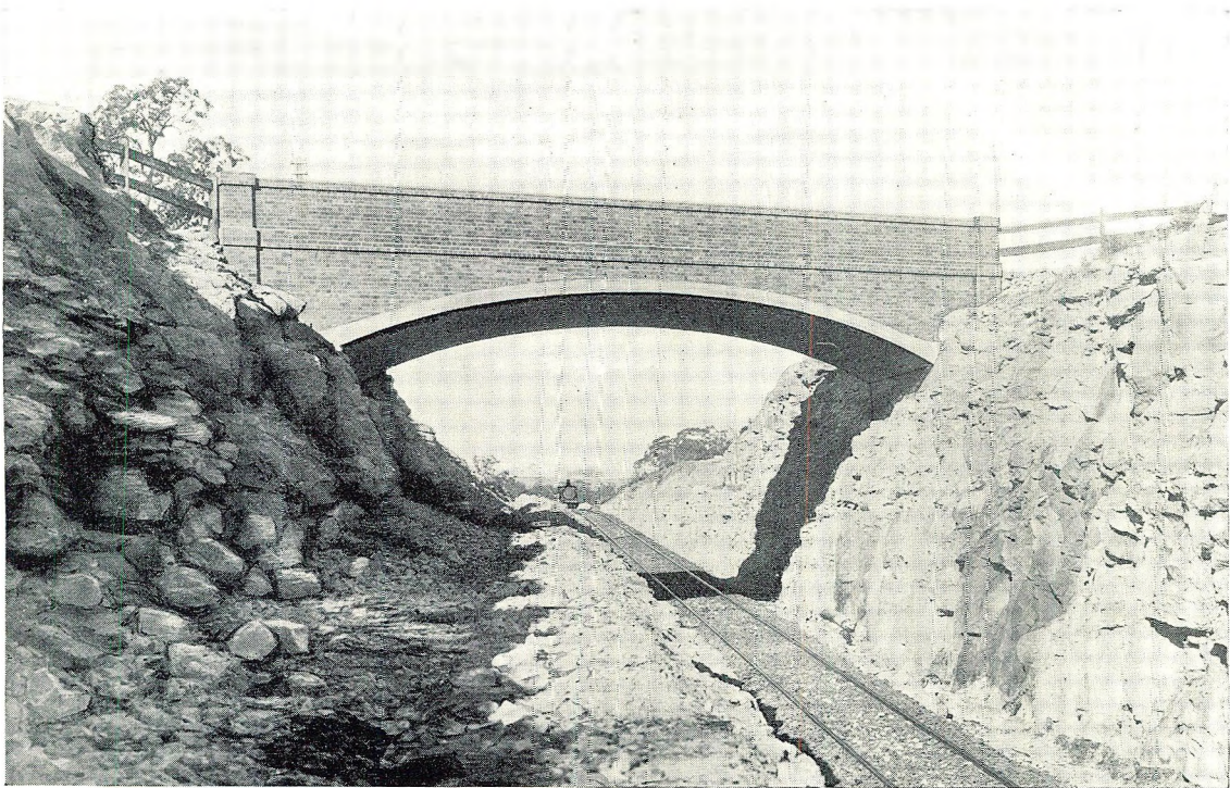
MAIN ROAD OVER BRIDGE. (MONIER ARCH.)
