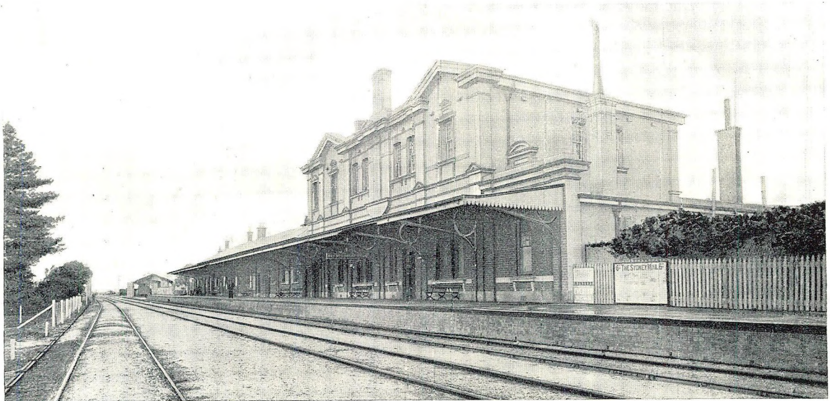
MAIN LINE STATION WITH REFRESHMENT ROOM.
