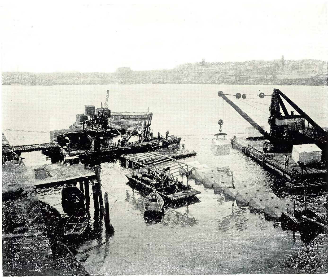
WHARF WALL ROUND DARLING ISLAND—SETTING CONCRETE BLOCKS.
