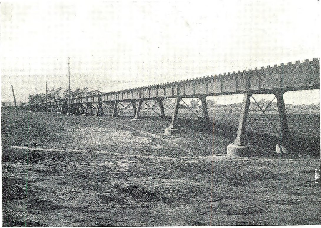
NEW STEEL VIADUCT.
