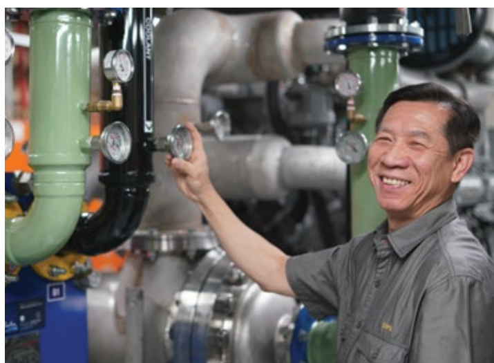
SAM TRUONG, BUILDING TECHNICIAN, MONITORS THE PERFORMANCE OF THE NEW GENERATORS.
