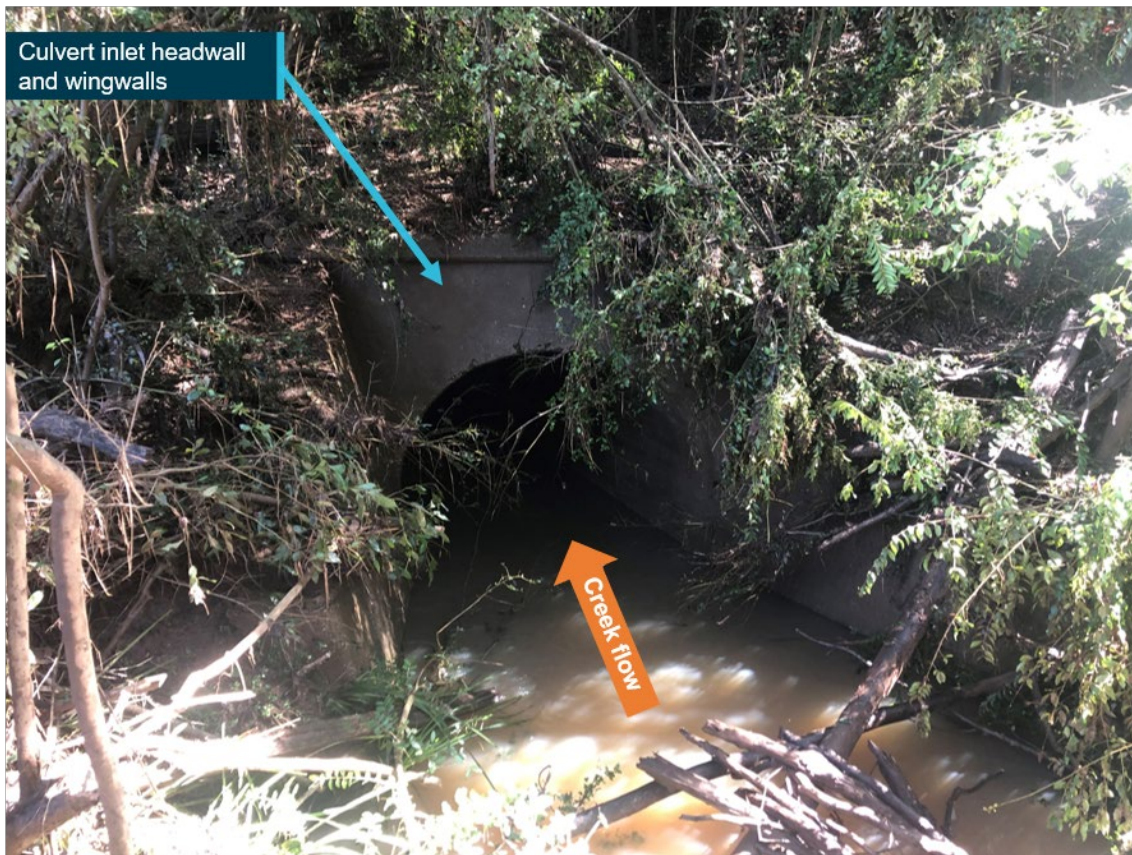
Figure 18: Culvert inlet
