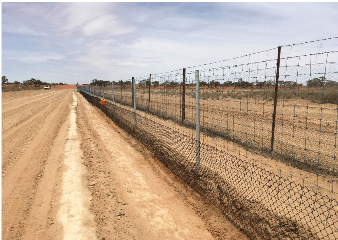
New section of fence under construction and old fence to be removed on completion.
