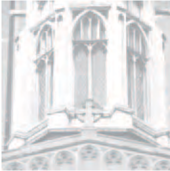
St Stephen's Uniting Church, Sydney. Photograph by Lianne Hall.
