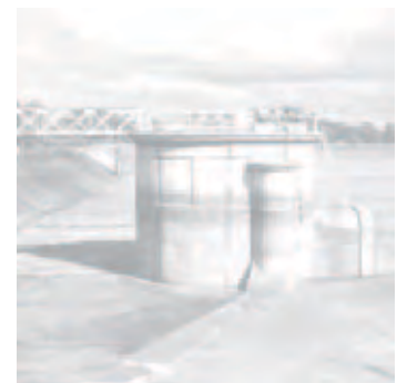
Potts Hill Reservoir, Yagoona. Photograph courtesy of Sydney Water Corporation.
