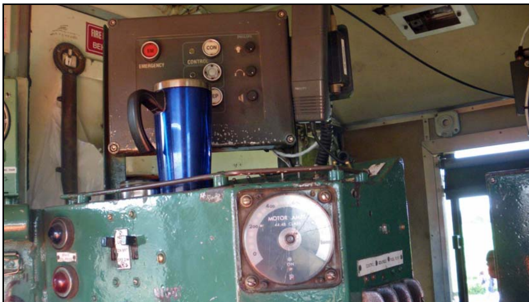
Photograph 9: Driver's cross cab view to the RMV approach direction
