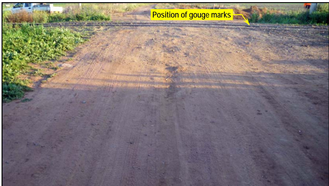
Photograph 13: Approach to crossing (Note no evidence of skid marks)
