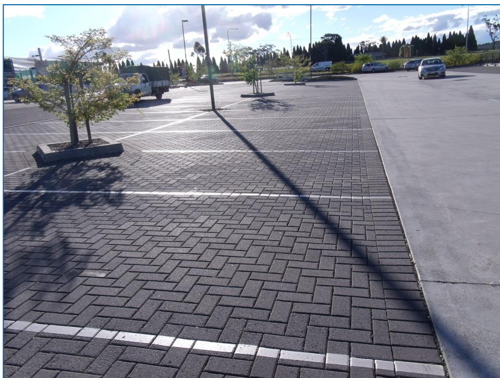
Figure C 3-9 Permeable pavement to harvest stormwater runoff at Bunnings
