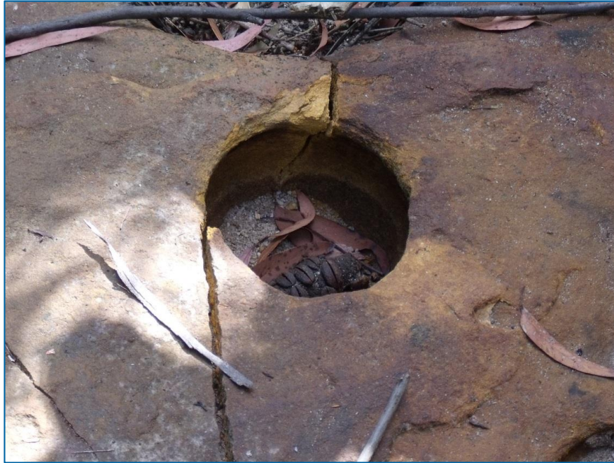
Figure C 3-14 Sandy Creek with creek bed cracking
