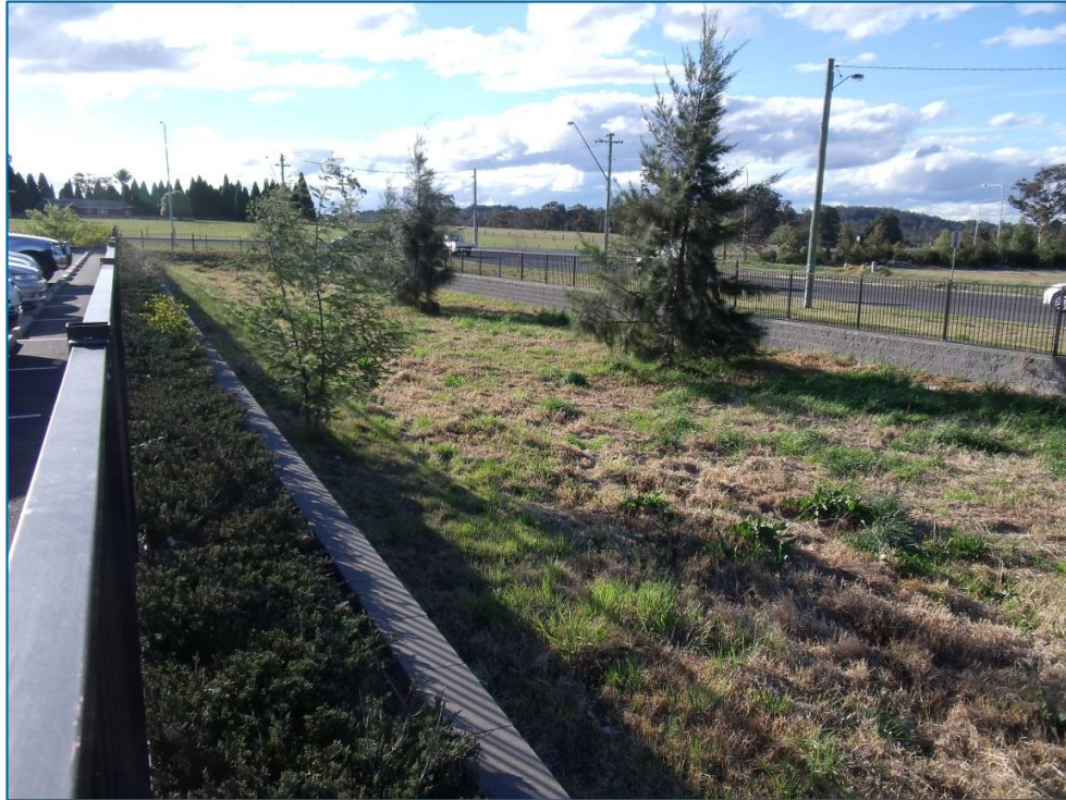
Figure C 3-10 Rain garden at Bunnings
