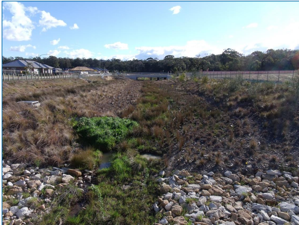
Figure C 3-8 Stormwater treatment Renwick estate
