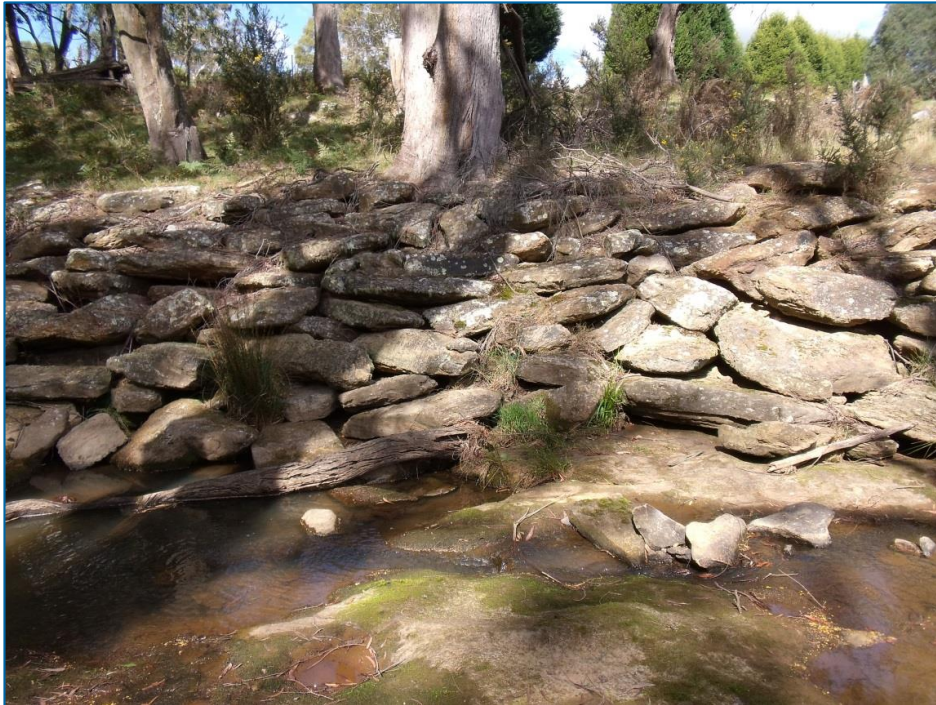
Figure C 3-2 Glen quarry creek bank works
