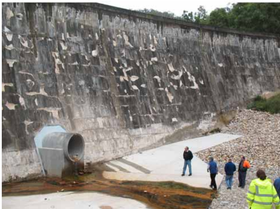
Redbank Creek Dam Partial upgrading works for this 16m high arch dam at Mudgee were completed in 2011. The DSC is currently working with various interested parties to finalise the upgrading of this dam.
