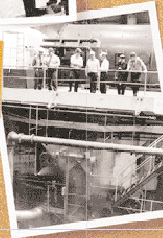
EXECUTIVE TEAM INSPECTION OF FIRE SUPPRESSION TESTING AT LIDDELL POWER STATION. TESTS ARE REGULARLY SCHEDULED DURING PLANNED UNIT OUTAGES AT LIDDELL AND BAYSWATER.
