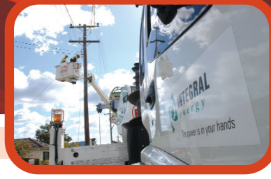
^ Pole replacement, Dapto
