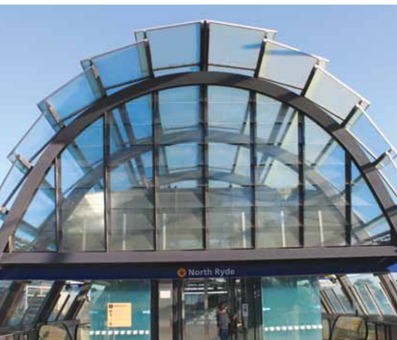
North Ryde Station is part of the Epping to Chatswood Rail Link.
