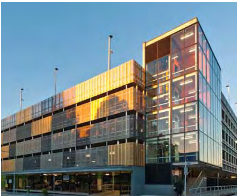
The new commuter car park at Revesby includes a range of security and accessibility features, including disabled parking, lift access, CCTV surveillance and lighting.
