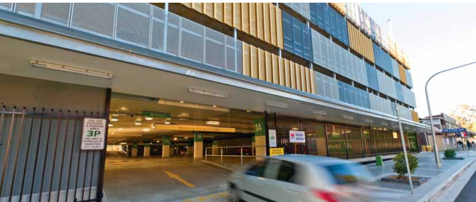
Revesby Commuter Car Park was completed in April 2011 as part of the Commuter Car Park and Interchange Program. It provides around 720 car parking spaces for commuters and shoppers.
