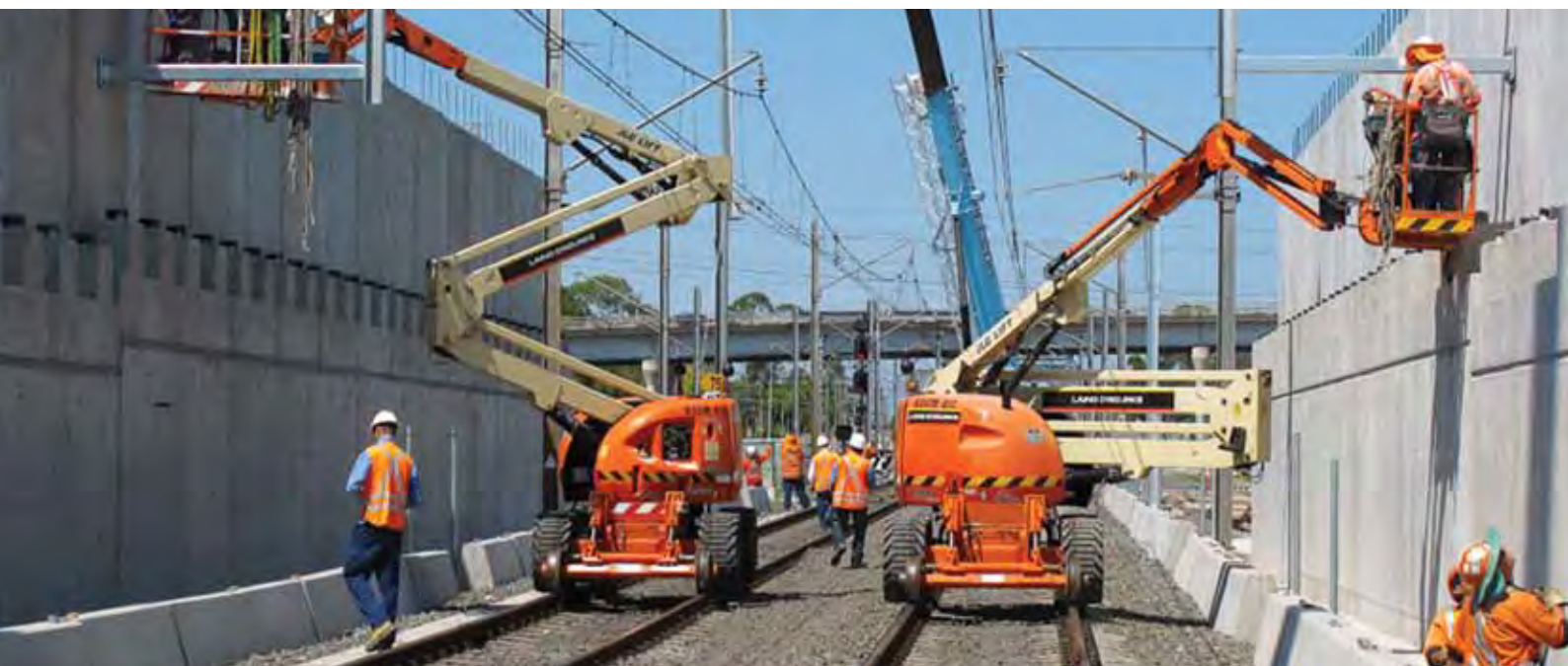
The northern flyover on the South West Rail Link.
