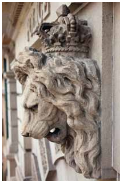
Stonework at 127 George Street, The Rocks
