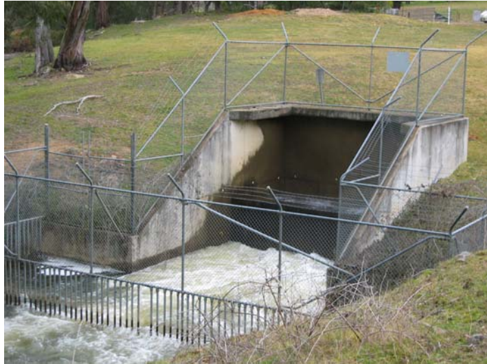
Figure 3.7 – Water released from Glen Quarry Cut into the Glen Quarry Creek, August 2003
