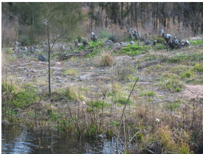
Figure 5.8 – Willow removal carried out by SCA along the Coxs River at Duddawarra Bridge, August 2003
