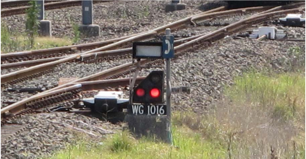
Photo 10: Close up of Signal WG1016 showing stop indication
