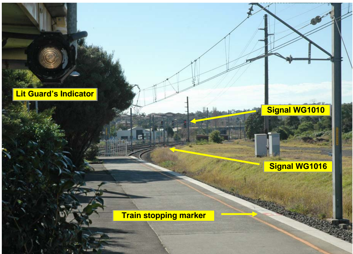
Photo 9: View of Guard's indicator (illuminated), stopping marker and signals visible from Unanderra platform
