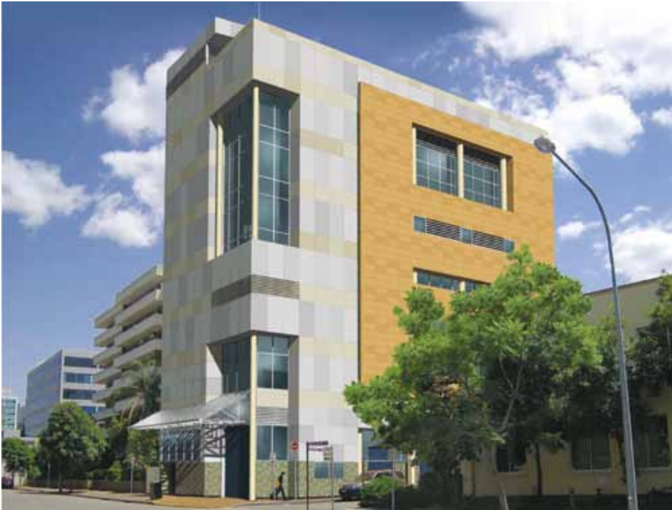
Giving Parramatta the power to grow – our $24 million East Parramatta Switching Station, designed to blend with the streetscape.
