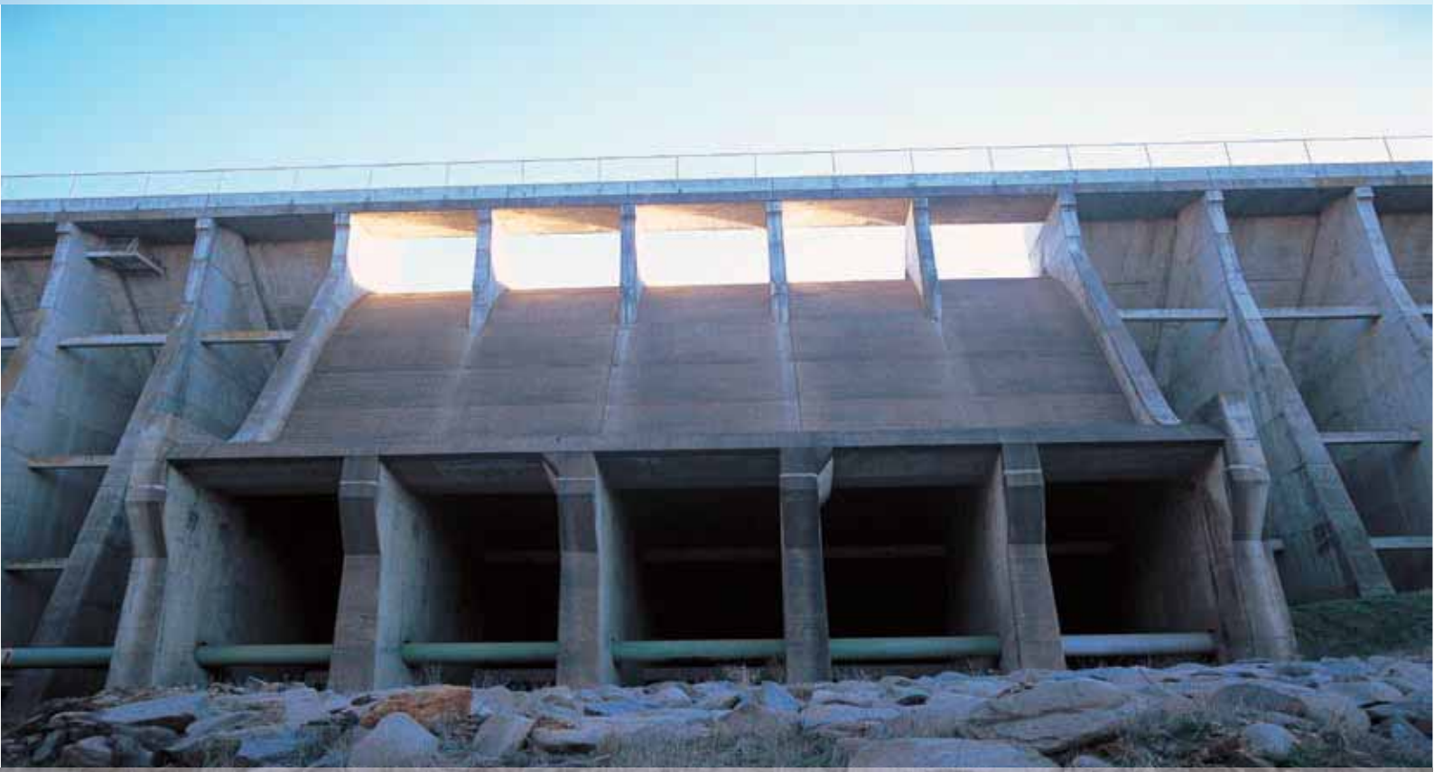
The dam wall at Oberon Dam.
