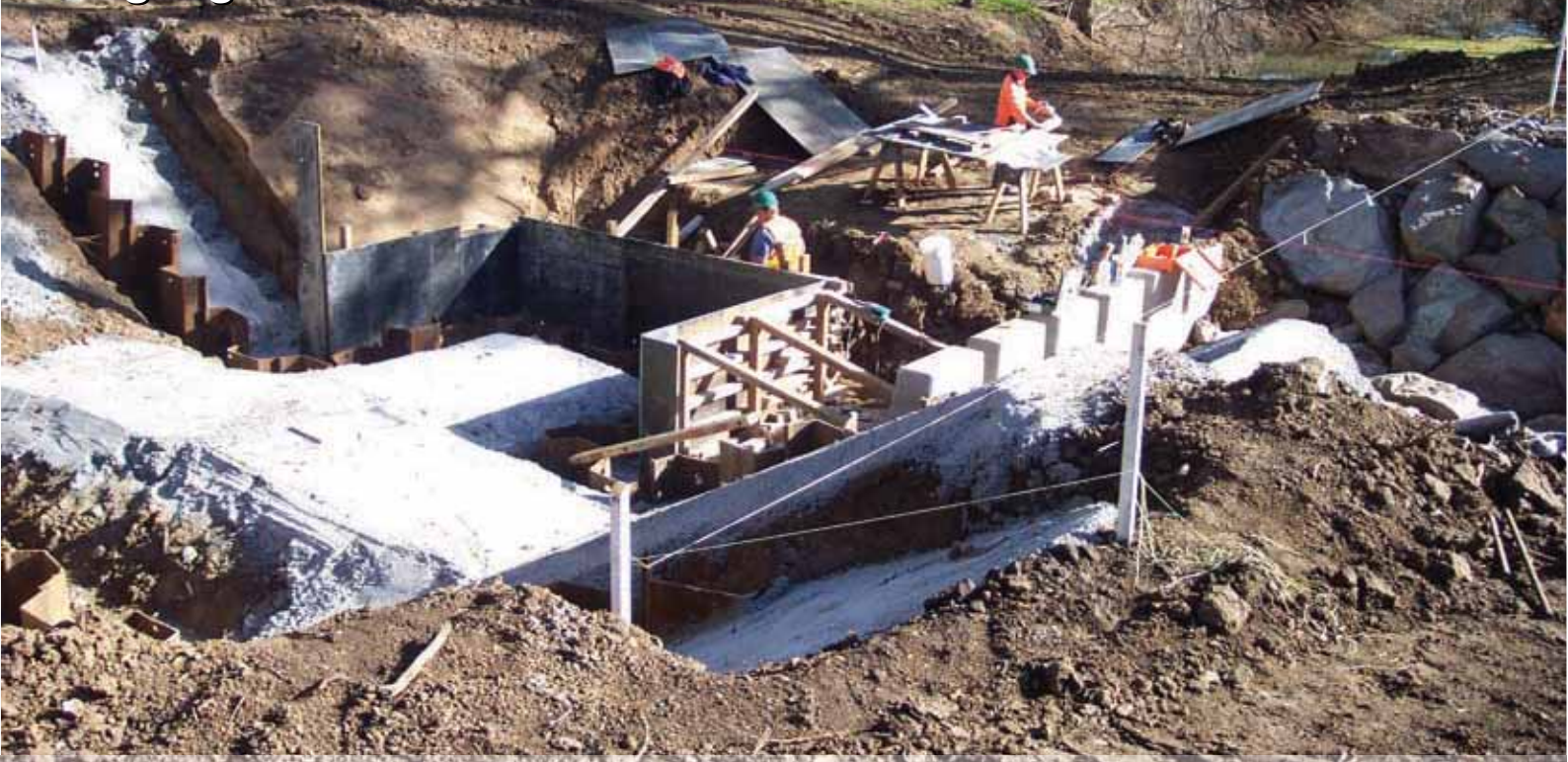
Construction of the innovative fishways for the Macquarie Weirs upgrade.
