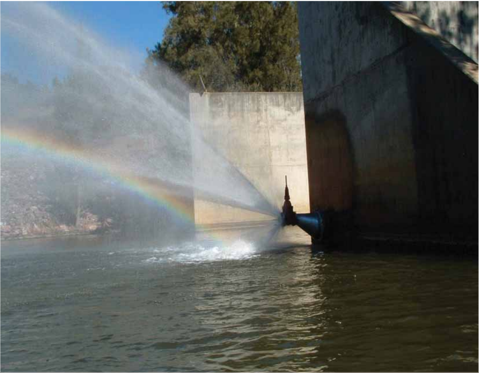
Chaffey Dam low level outlet penstock.
