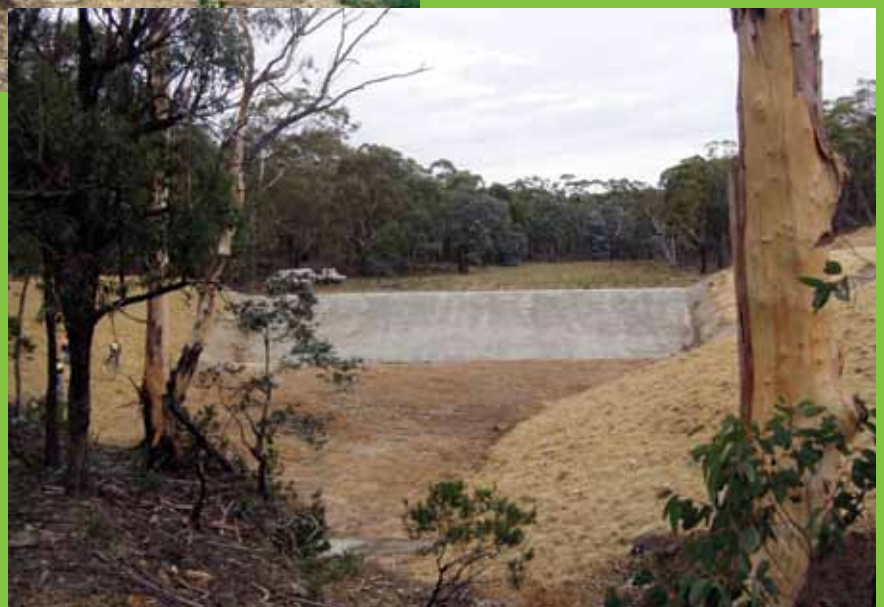
AFTER Long Swamp, Junction Creek works showing a flume constructed to stop the gully head cut
