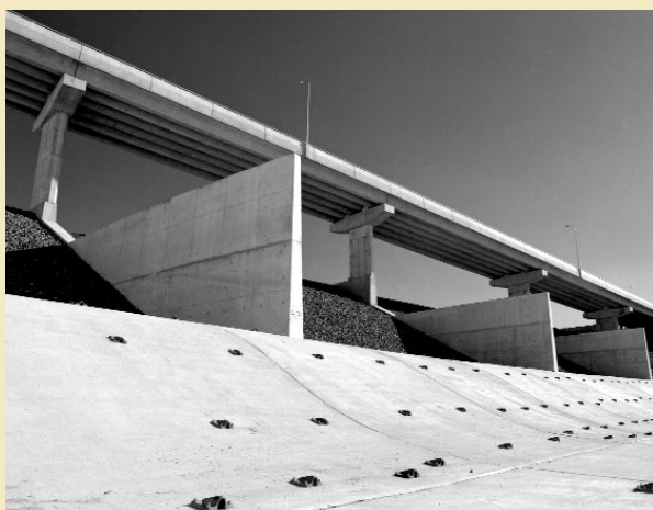
Warragamba Dam Auxiliary Spillway
