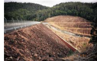
Clarrie Hall Dam
