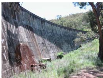
Redbank Creek Dam
