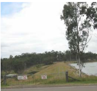
Drayton Mine Water Supply Dam
