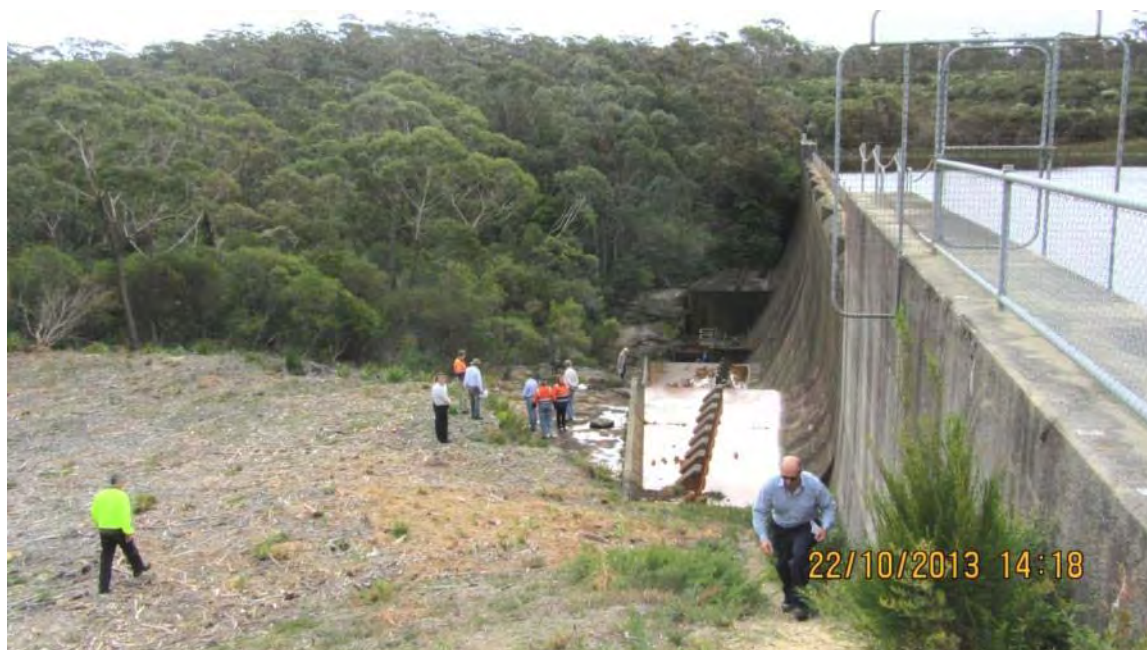
Porters Creek Dam. DSC members and staff inspected this 17m high post-tensioned concrete gravity dam in October 2013 in conjunction with a DSC country meeting.
