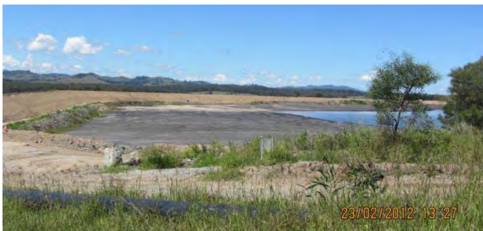
Camberwell Tailings No. 2 Dam. Initially constructed in 1995, this earth and rockfill dam has risen to 33m high and now has a storage capacity of 5,300ML. It stores coal tailings from Integra Coal Operations in the Hunter Valley.
