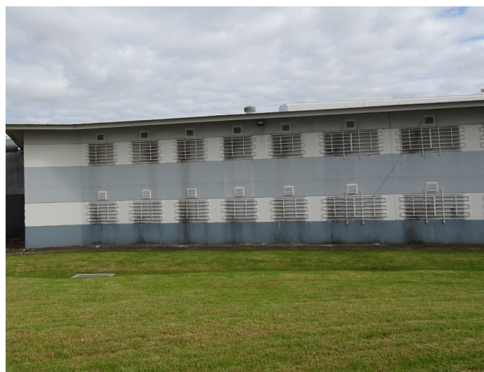
Fordwick accommodation block
