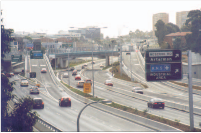
Looking west along the widened and reconfigured Gore Hill Freeway at the rebuilt Reserve Road overpass in Artarmon, 25 March 2007.
