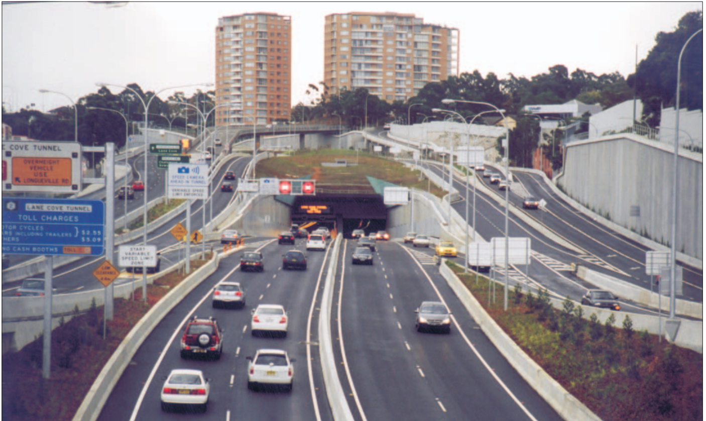
Looking west from the rebuilt Reserve Road bridge over the Gore Hill Freeway in Artarmon towards the eastern portals of the Lane Cove Tunnel, 25 March 2007.
