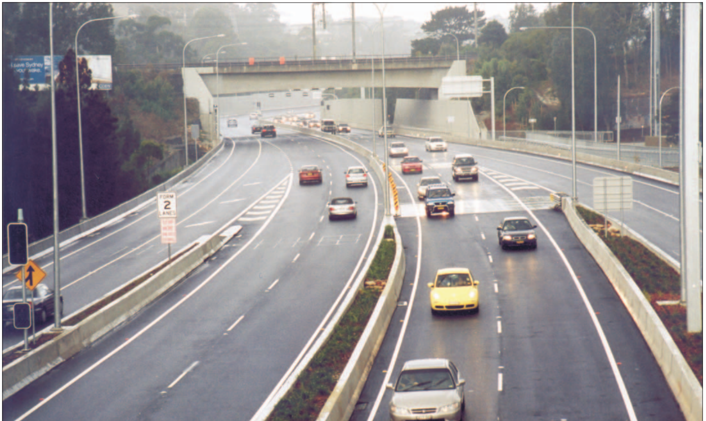
Looking east along the widened Gore Hill Freeway under the North Shore railway line bridge in Artarmon, 25 March 2007.
