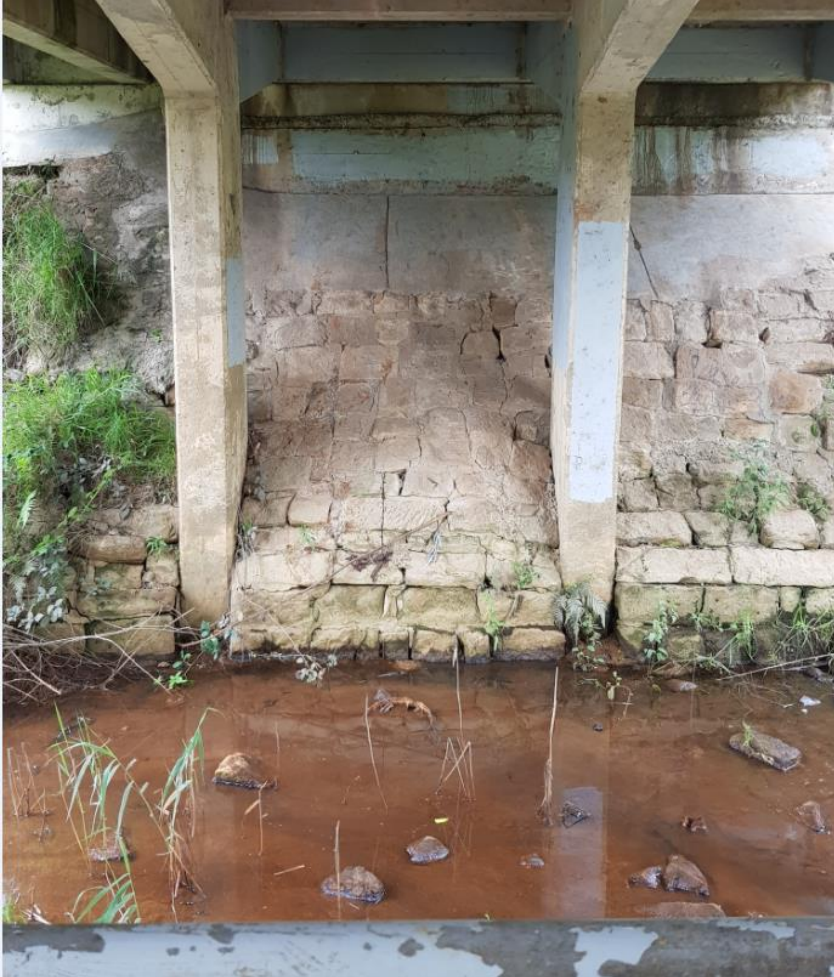
Figure 4: Red sludge is an indicator of Acid Mine Drainage arising from the high sulphur content of coal/rock 10
