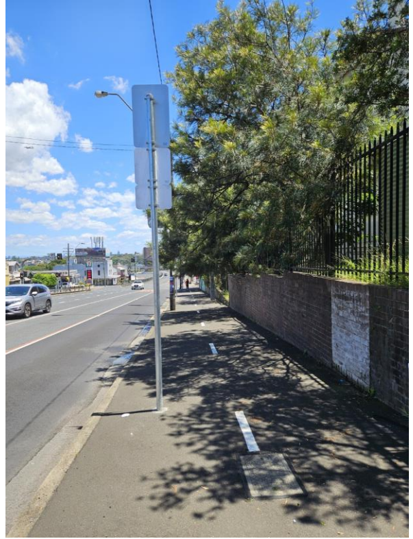
Approaching Darling St. Example of dangerous pole placement, in the middle of shared path downhill lane. Needs to be removed urgently.
