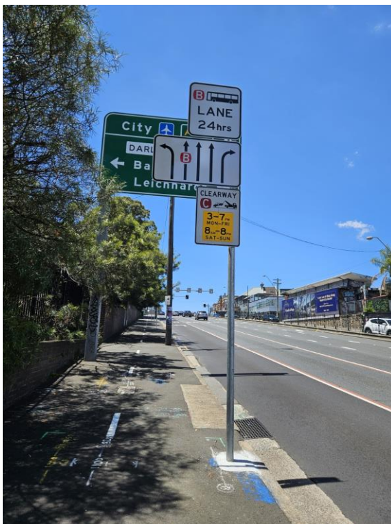
Just past Wellington St. Example of better pole placement as it is at the side of the lane. However, the pole does not have reflective markings, and pole was not actually required as the existing pole supporting the green directional signage could have been used.
