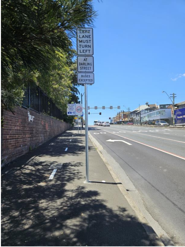
Approaching Darling St. Example of dangerous pole placement, in the middle of shared path downhill lane. Needs to be removed urgently.
