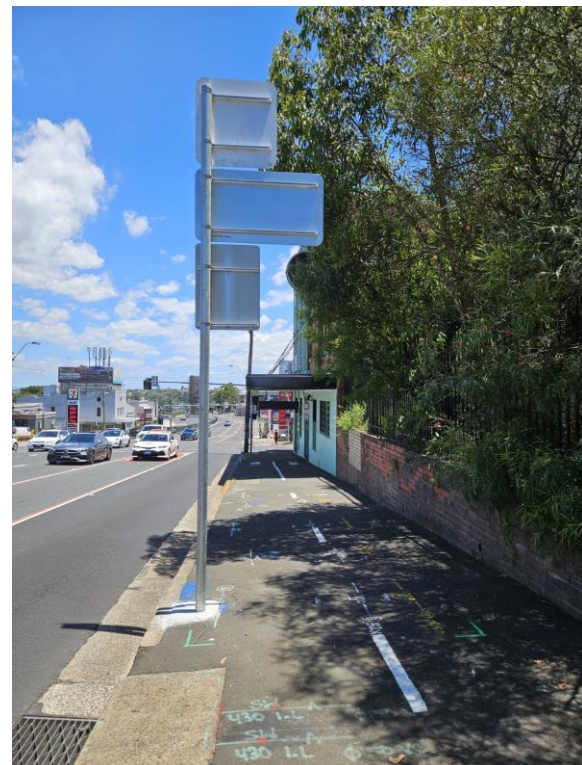
Just past Wellington St. Example of better pole placement as it is at the side of the lane. However, the pole does not have reflective markings, and pole was not actually required as the existing pole supporting the green directional signage could have been used.
