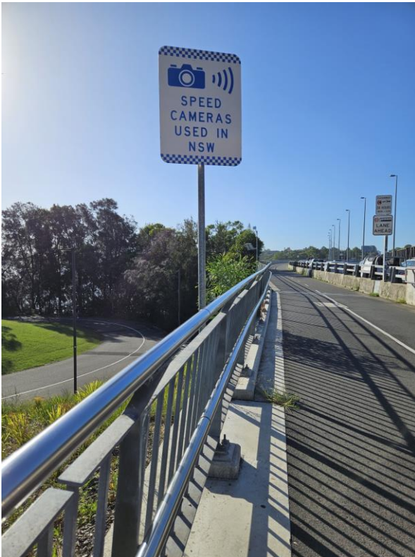
Start of Iron Cove Bridge. Example of acceptable pole placement – pole is behind railing.
