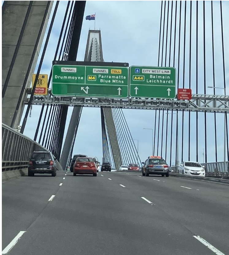
Figure 8 9: Misalignment of overhead arrows and lanes
