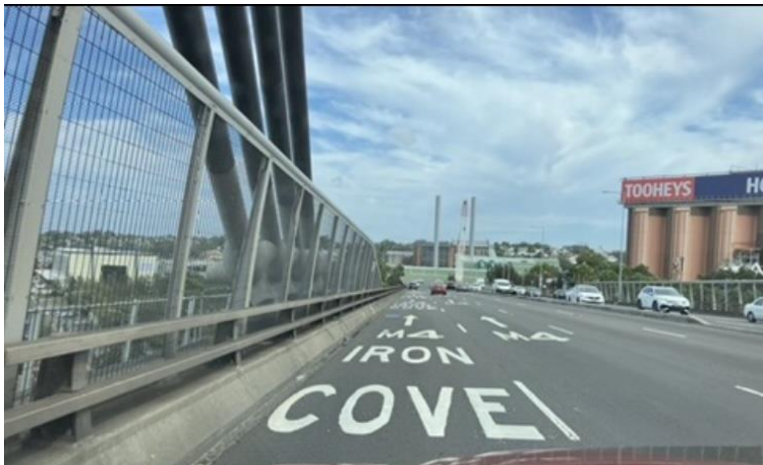
Figure 9 10: Road marking does not use the same names as the previous overhead sign
