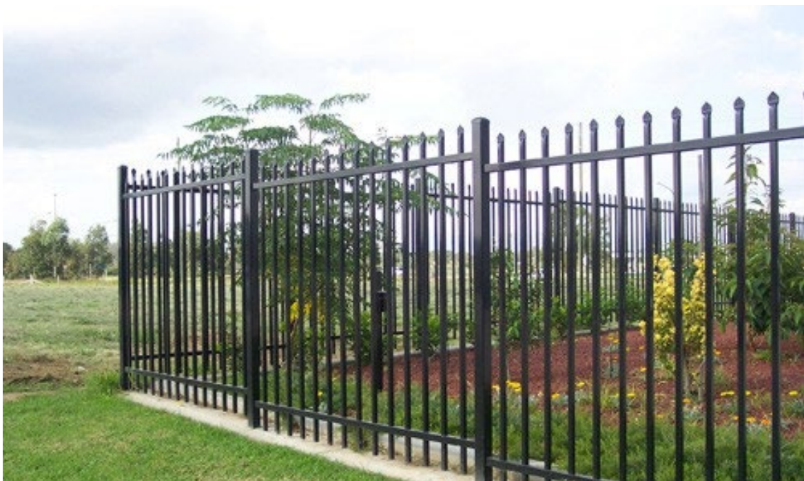
Figure 1 : Example of welded tube panel design security fence.
