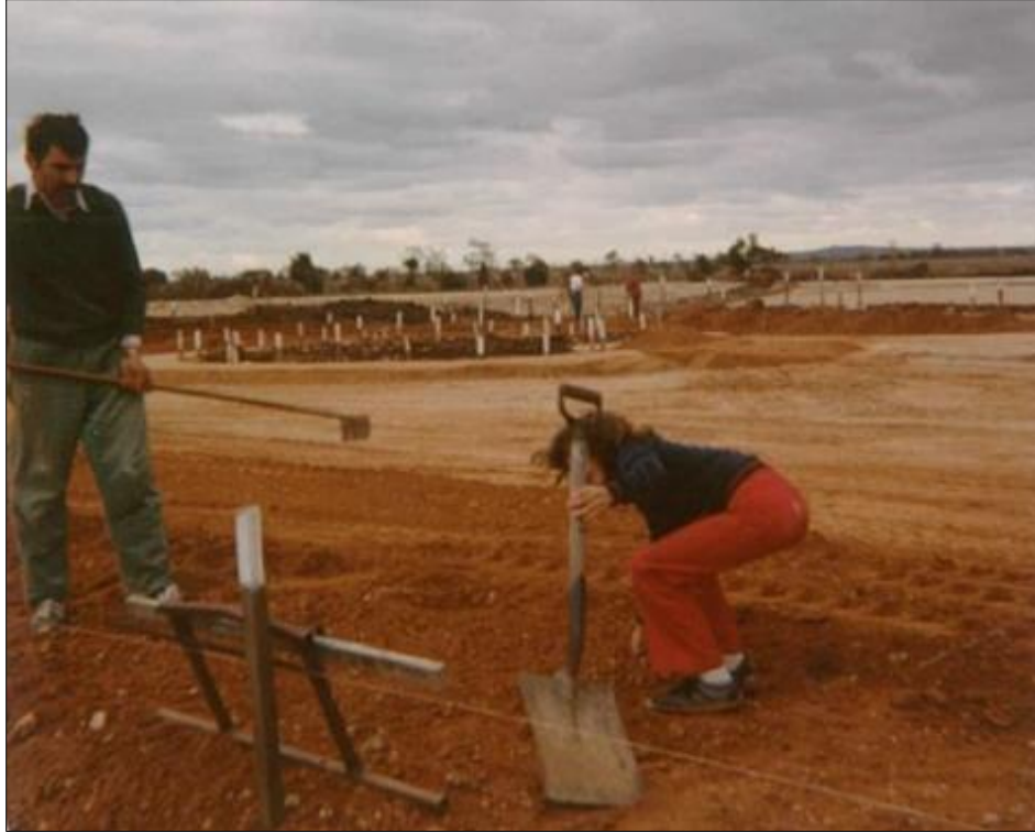
Figure 2: Larissa Kaput (child in foreground) working on the construction at Melton Assembly Hall
