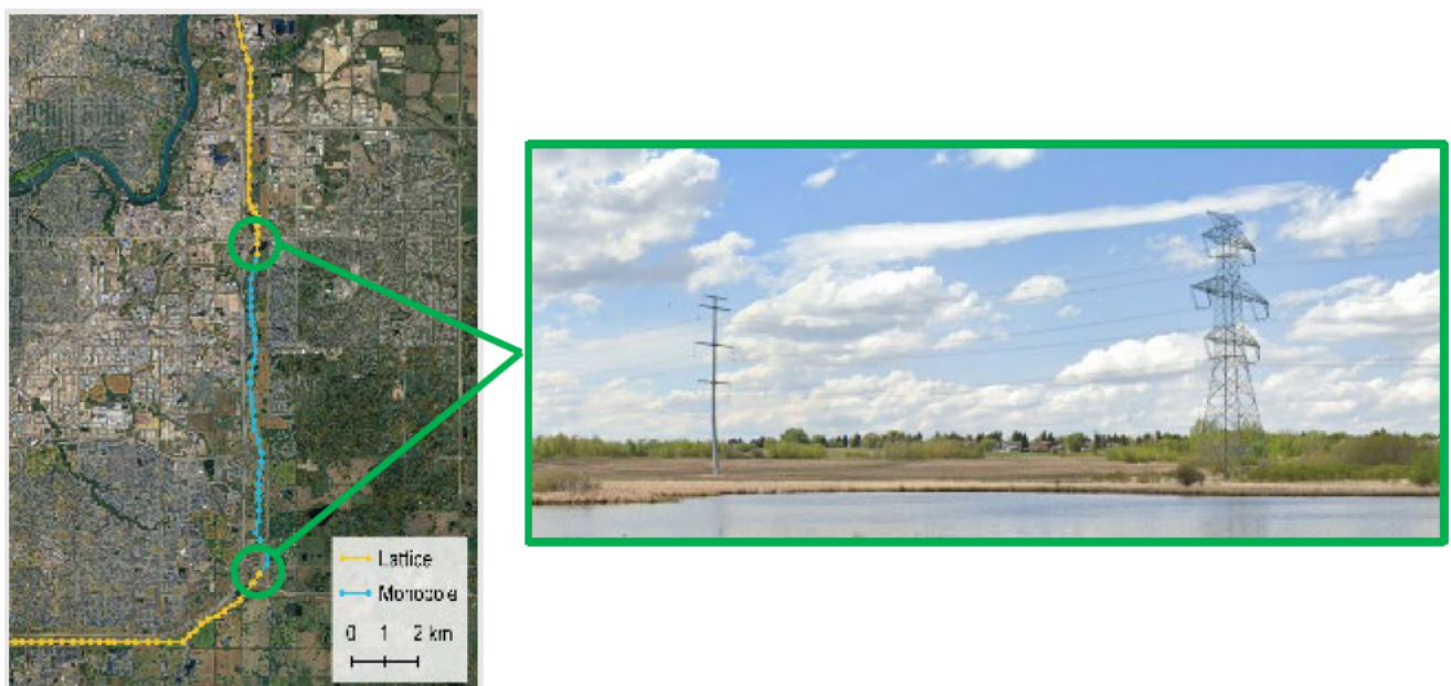
Figure 1. Monopoles used in 10km of transmission line to gain community support.
