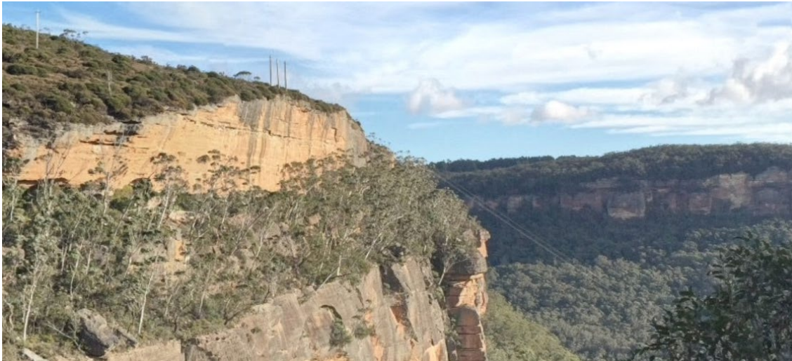
Figure 7: Overhead lines at Shipley Plateau, Blackheath spanning a 100m escarpment 22
