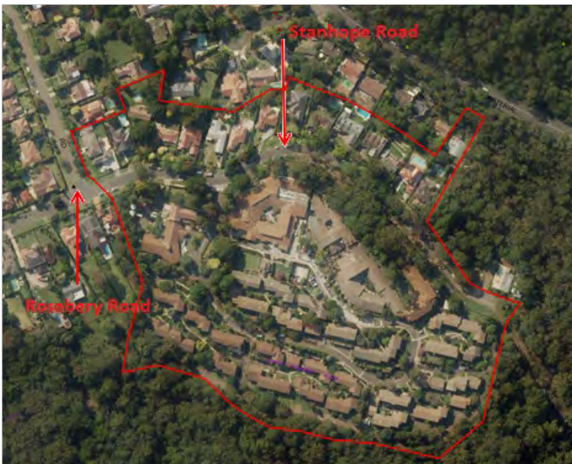
Aerial Photo – Outline showing Catchment Area for Assessment of Bushfire Evacuation Risk
