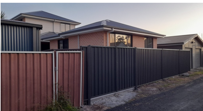
Umina townhouses with tin fence hard up against the back room and on a rear landway – no room for any plants.
