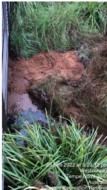
Figure 2: Tempe Recreation Reserve showing cork infill and plastic turf seeping into the Cook's River after a high rainfall event. This field includes a surrounding curb designed to prevent microplastic loss and overland runoff.
