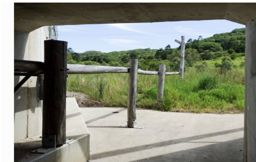
Wardell Road Underpass , Pacific Highway, Wardell
