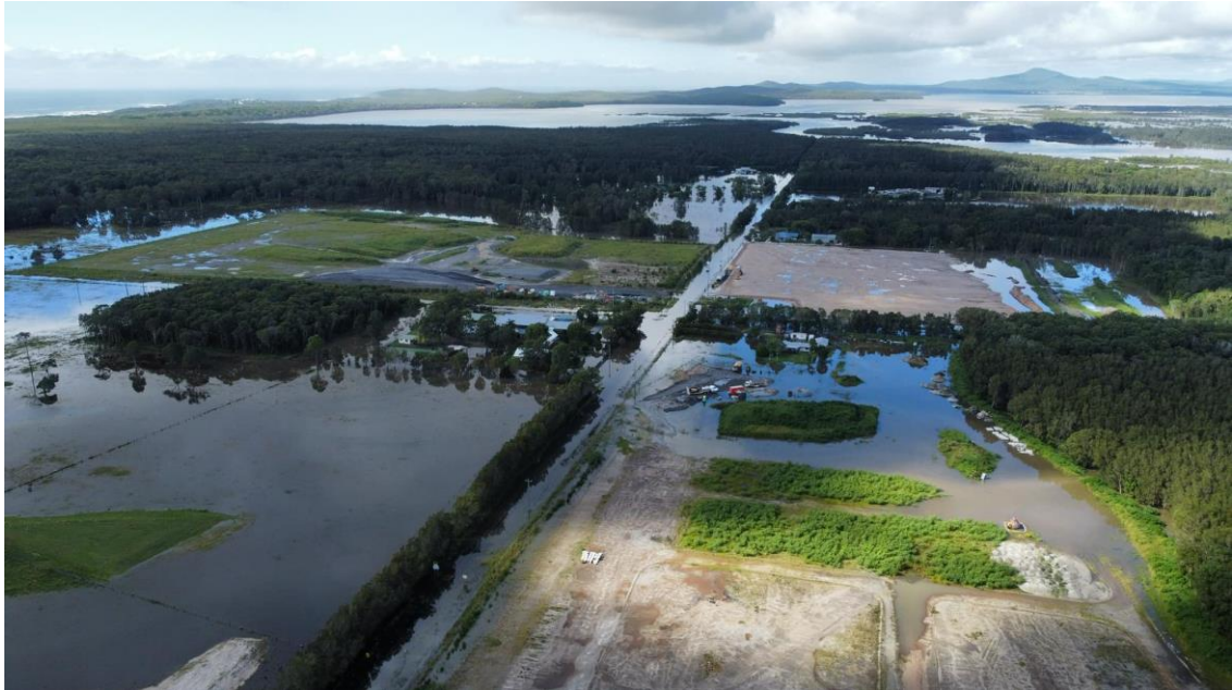
March 2022 Carrs Drive west Yamba flawed flood plain planning result with fill
