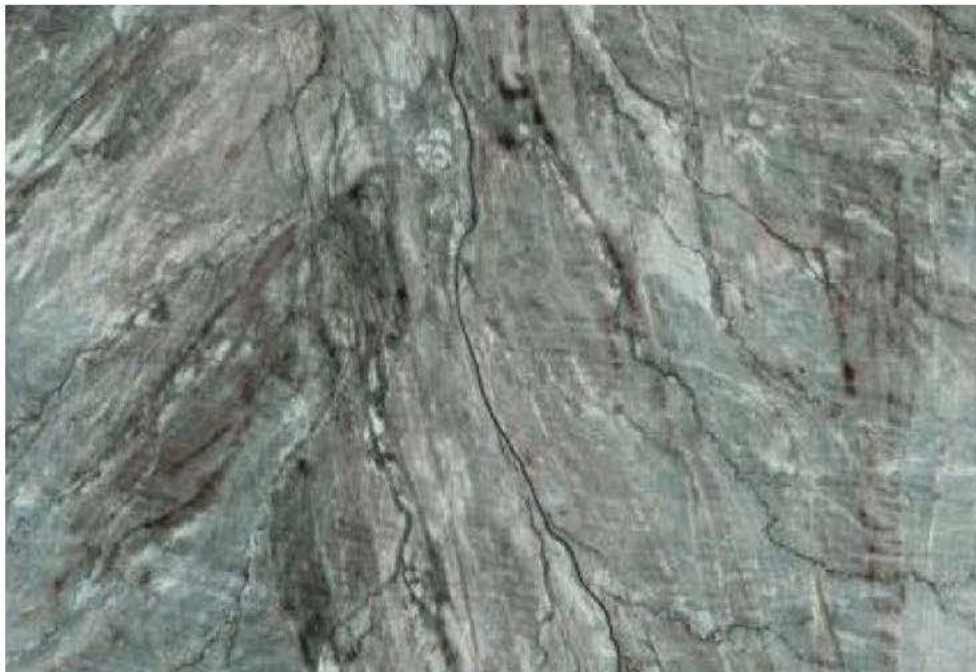
Soil erosion creating gullies on the southern tailings dam as seen from Google earth.
