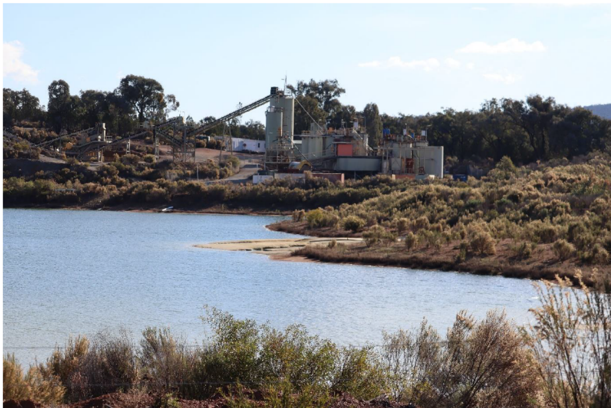
Photo 5 Broula King TSF dam - northern section. The TSF should not hold water but dry material from the mining process. The lack of water management on site has created a small lake of contaminated water. Photo taken 10 July 2021, but the TSF looks the same in August 2023.
