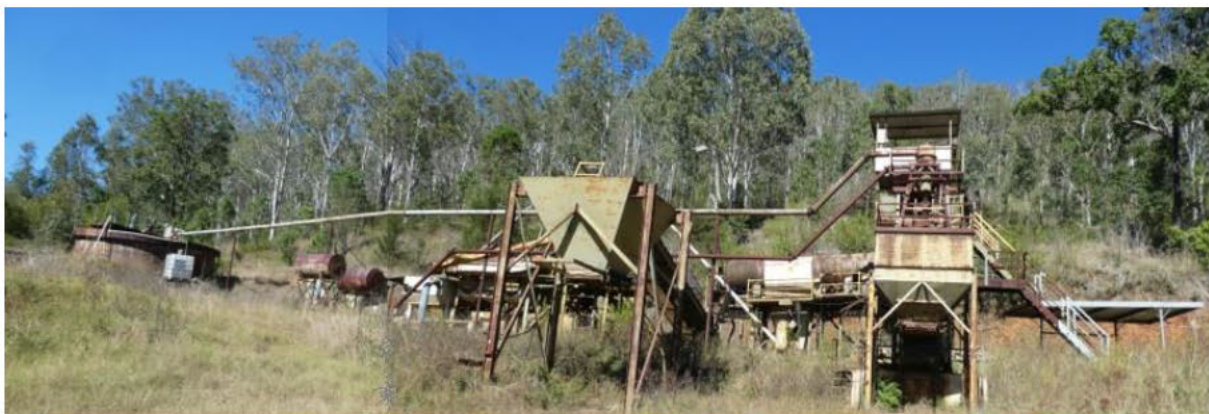
The wash plant today, a rusting relic and eyesore, typical of other sites across the country and now set to reopen to mine material on site, and also process material sourced under a separate exploration licence.
