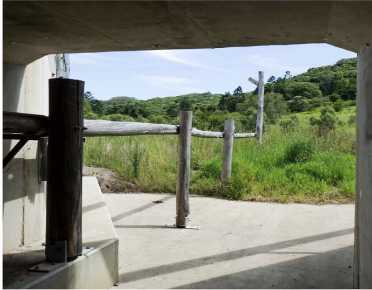
Wardell Road Underpass , Pacific Highway, Wardell
