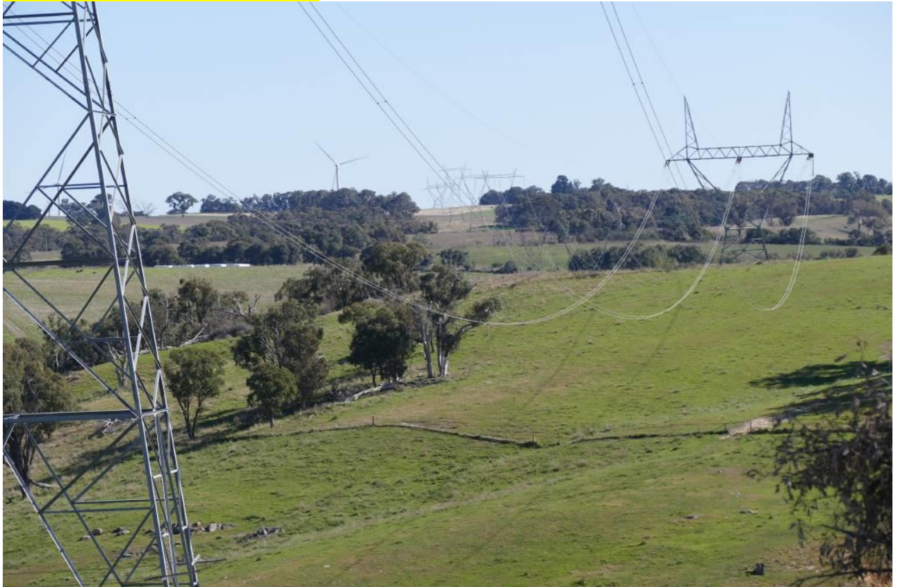
(Rows of transmission towers near Crookwell, southern NSW)
