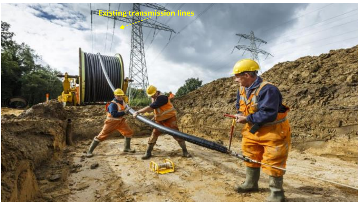
Figure 3. Underground transmission line being installed within existing transmission easement. Source: Renewables Grid Initiative
