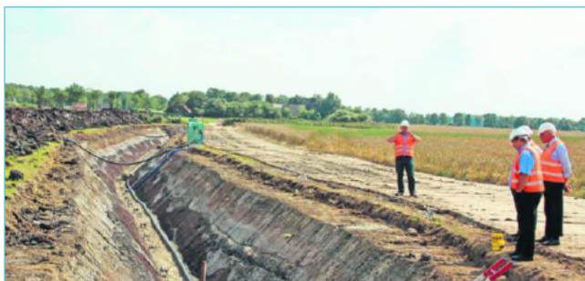
525kV HVDC cable trench
