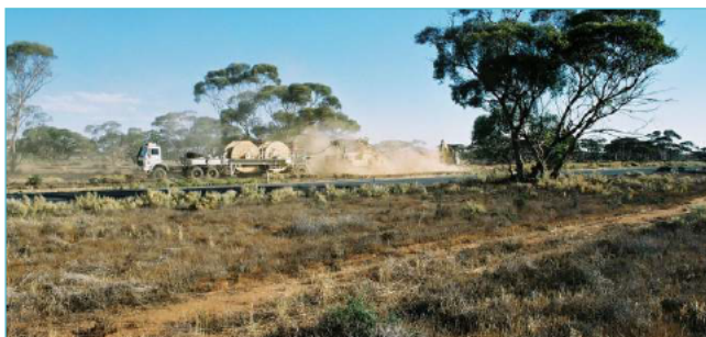
Underground co-location development using a Vermeer T755 Chain Trencher
