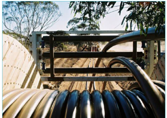
Installation of underground HVDC cable
