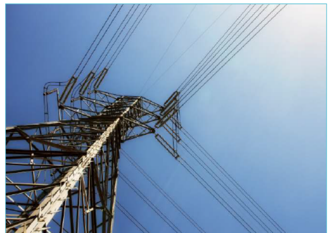
Installation of HVDC cable on existing HVAC overhead infrastructure
