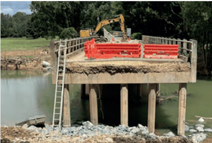
Figure 15: The bridge on Main Arm Road between Mullumbimby and Main Arm, showing a large section washed away by the Brunswick River two weeks earlier. (Photo courtesy of Risk Frontiers 2022)
