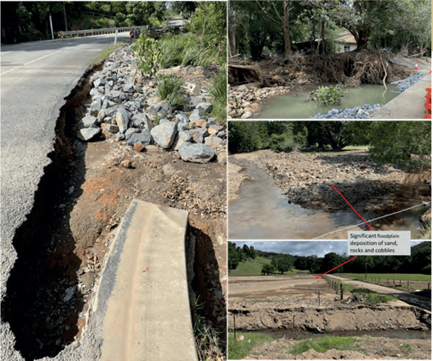
Figure 17: Road base and soil erosion from roadways and tree roots (left & top right) and evidence of fluvial geomorphic change with the deposition of sand, rocks and cobbles on floodplains (mid and bottom right) caused by deep and fast flowing flood waters in the confined Brunswick River catchment between Main Arm and Upper Main Arm. (Photo courtesy of Risk Frontiers 2022)
