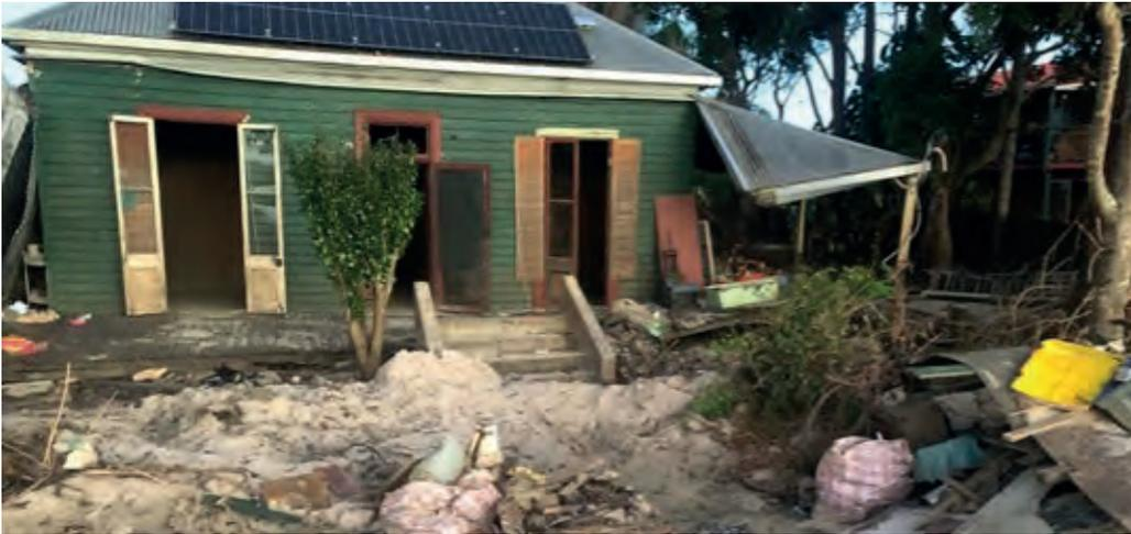
Figure 10: Broadwater residence showing structural damage and large amounts of flood-deposited sand in the front yard. (Photo courtesy of Risk Frontiers 2022)
