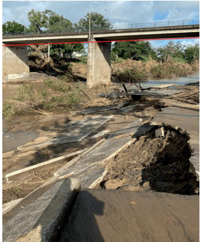
Figure 3: The Richmond River in Casino beneath the Irving Bridge. Red line indicates the approximate peak height of flooding on the 27th of February. Note the destroyed roadway and trees lain over by the force of flood water. (Photos courtesy of Risk Frontiers 2022)
