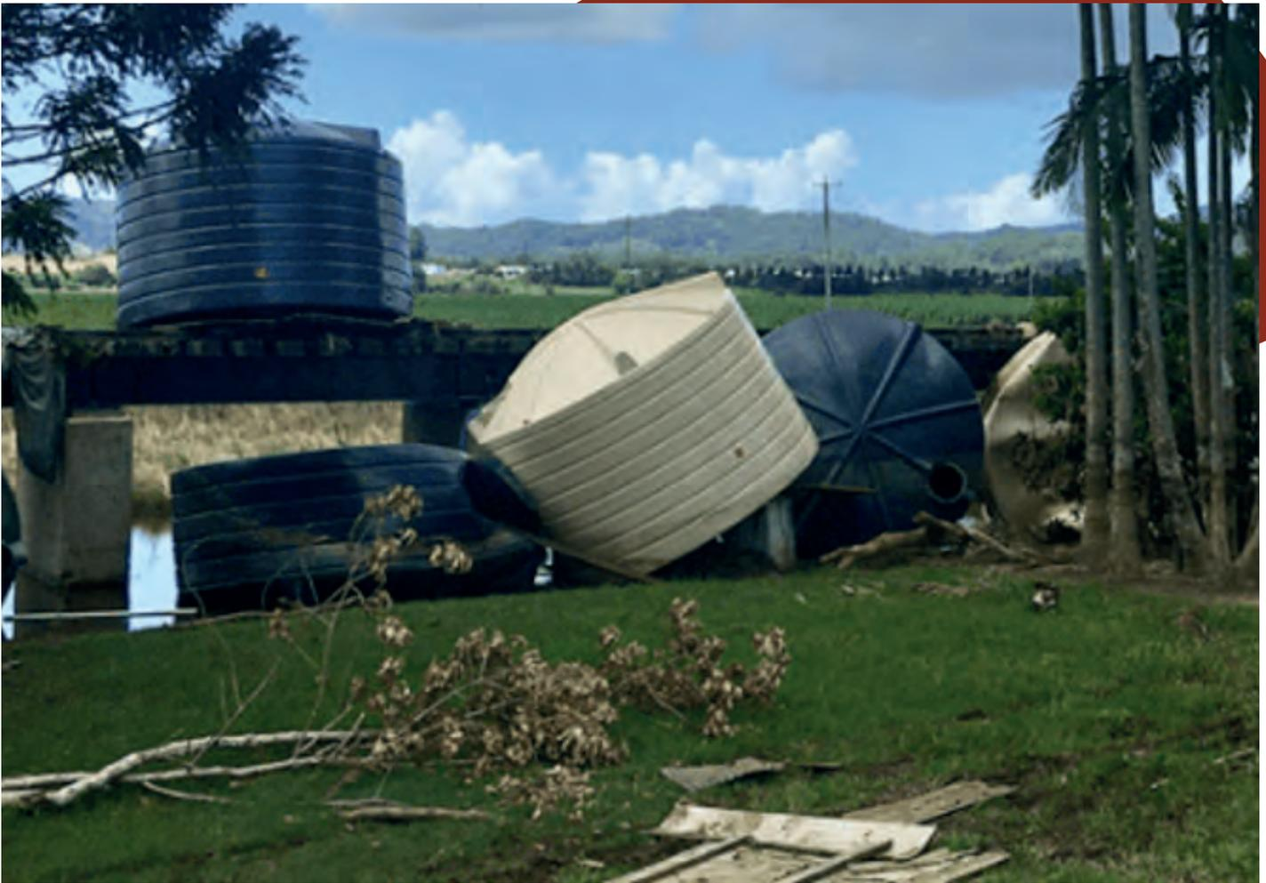
Figure 14: Plastic water tanks are easily transported by flood waters as seen in this example from South Murwillumbah where a number have been forced beneath a railway bridge. (Photo courtesy of Risk Frontiers 2022)
