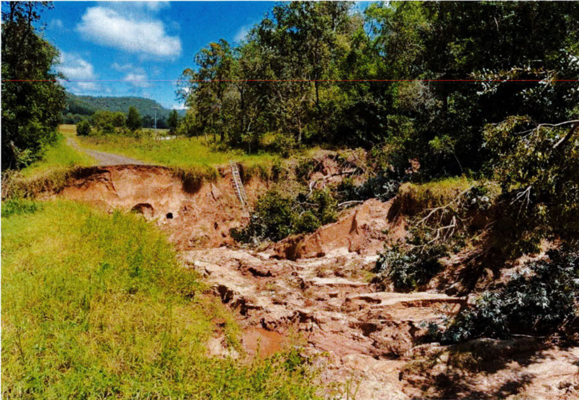
Council is facing more than $100m in major road repairs following the floods. This washaway on Upper Cherry Tree Rd, Mongogarie left residents isolated.
