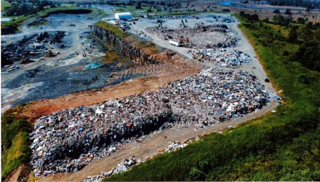
Waste from the flood clean-up was stored at Council's quarry in Coraki until it could be transferred to external disposal sites. Some 80,000 tonnes of waste (six times our community's annual contribution to landfill) was collected after the flood.
