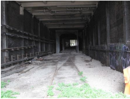
Tunnel under Railway Square
