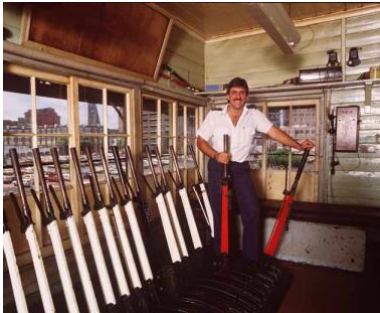
Interior of Ultimo signal box c1984
