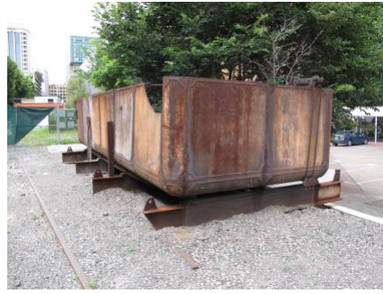
Water tank, ex-West Shed, Sydney station
