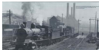
Goods train, Ultimo Road bridge 1950 (SRO)
