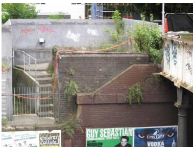
Brick foundation for Ultimo Street signal box
