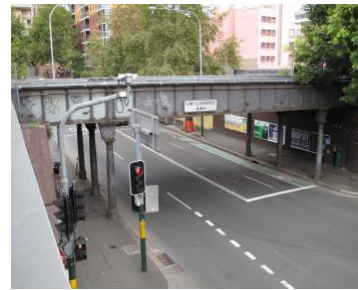
Ultimo Road wrought iron bridge
