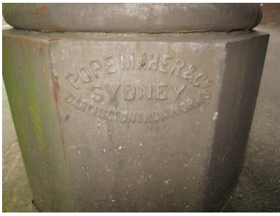
Cast iron columns, Ultimo Road bridge
