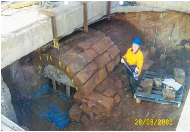
Excavating stone & brick culvert, 2003
