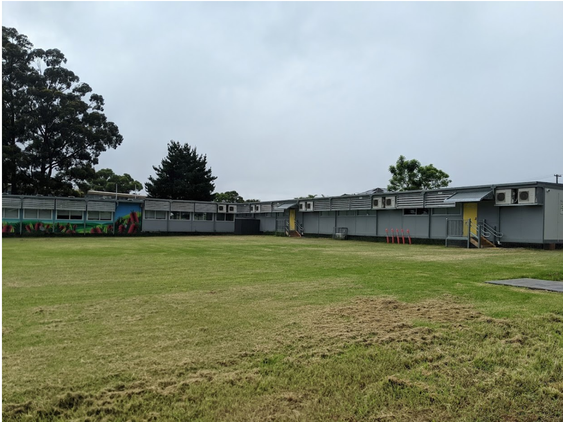
Figure 10 – Demountables at Picnic Point High School (author’s own photo)
