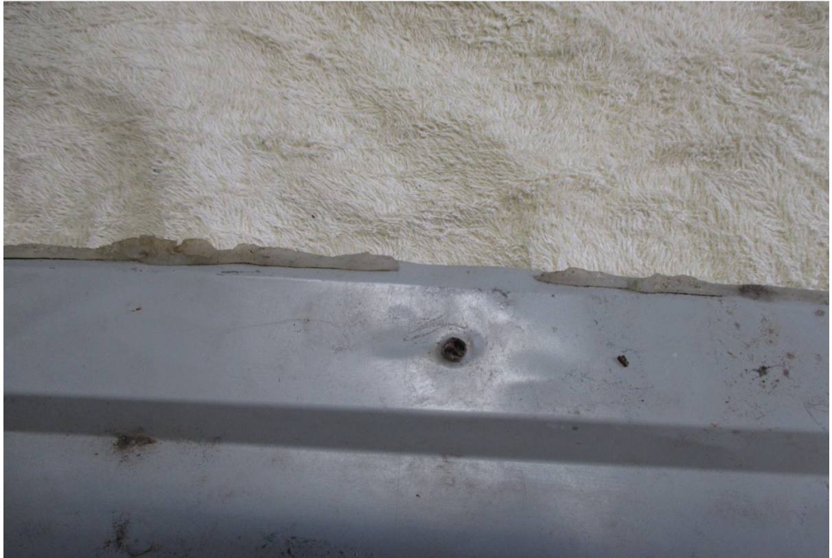
Close up of the glue edge to attempt to provide waterproofing with the brick surfacer
