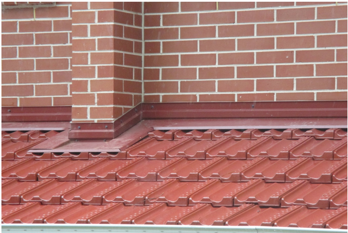
The same example photo of bad roof design as detailed in the previous submission. No flashing or damp course was used and lengths of pressed steel sheet were glued to the wall to cover the gap.
