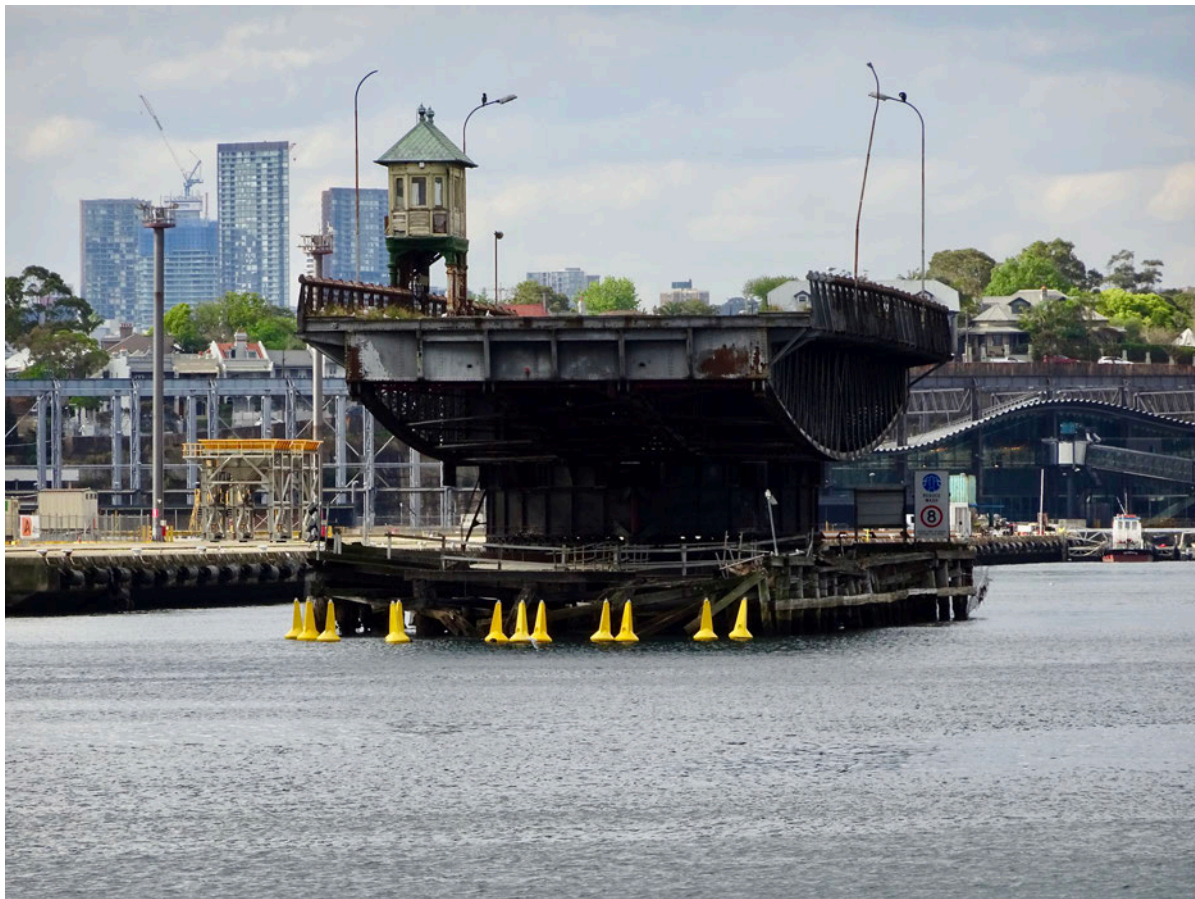
Image of Glebe Island Bridge courtesy of Phil Vergison
