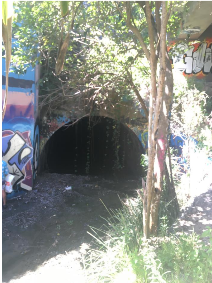
Image #4: Storm Water Tunnel West
