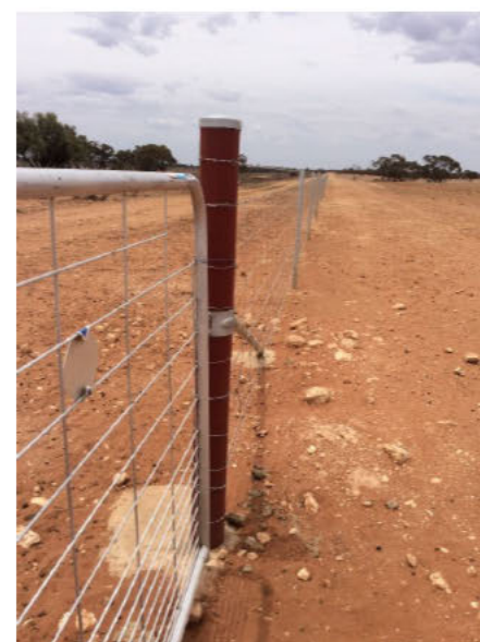
Figure 2: Semi-exclusion fencing being erected at Kerribee Station to help manage kangaroo impacts
